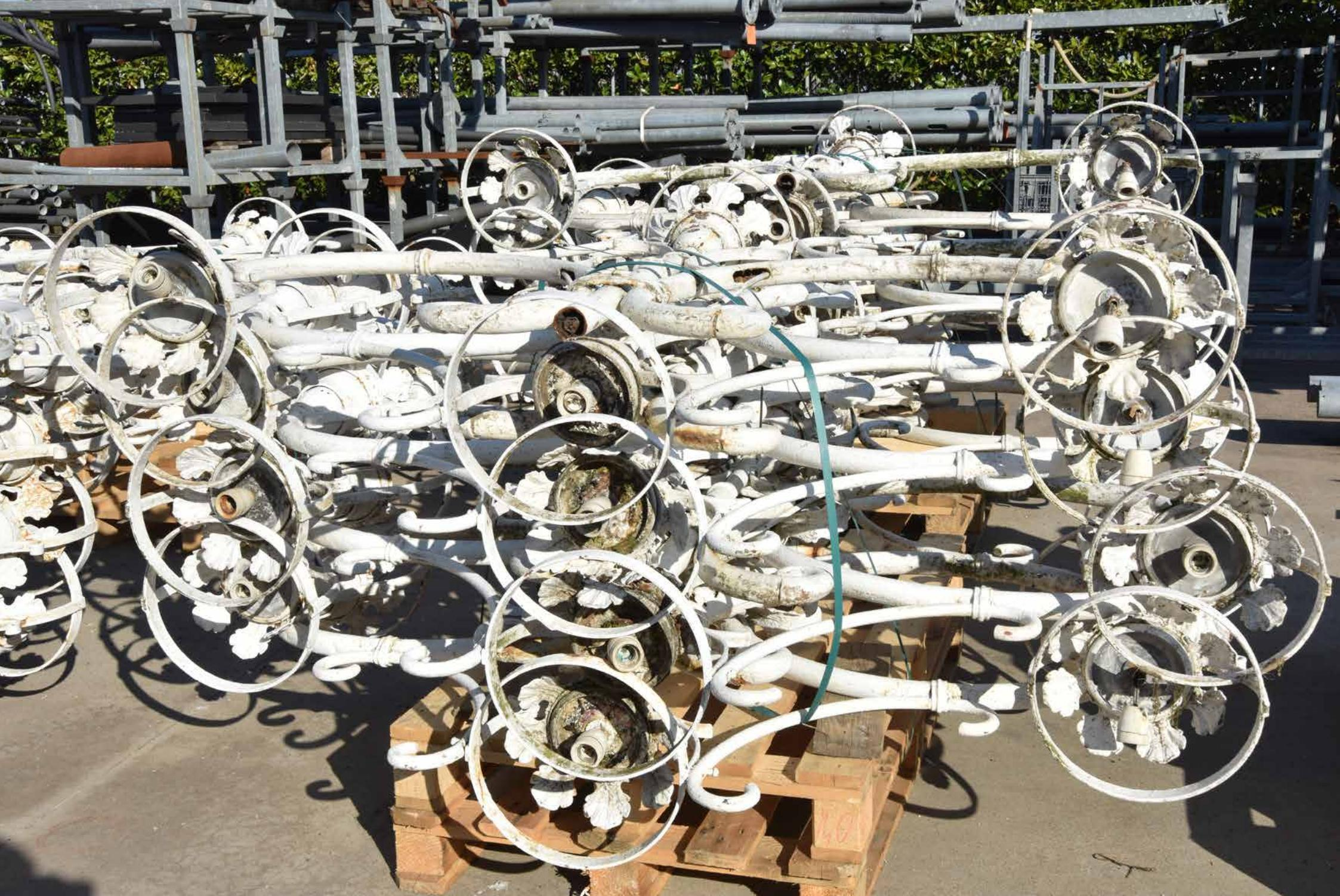
Neri has now restored the 50 original lamp posts, cleaning them to distinguish between integral and damaged parts. Each item saved has been catalogued and restored, integrating it where necessary with specially made identical elements.
