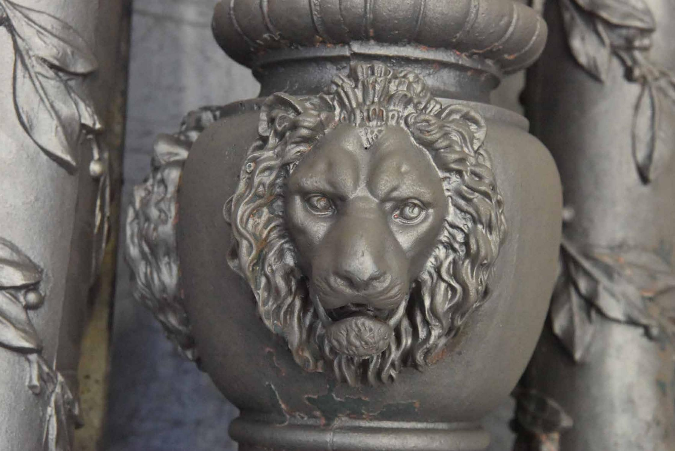
All of the individual elements recovered after disassembly were counted and, after being cleaned, were re-welded, recomposing the original look of the lamp post.
