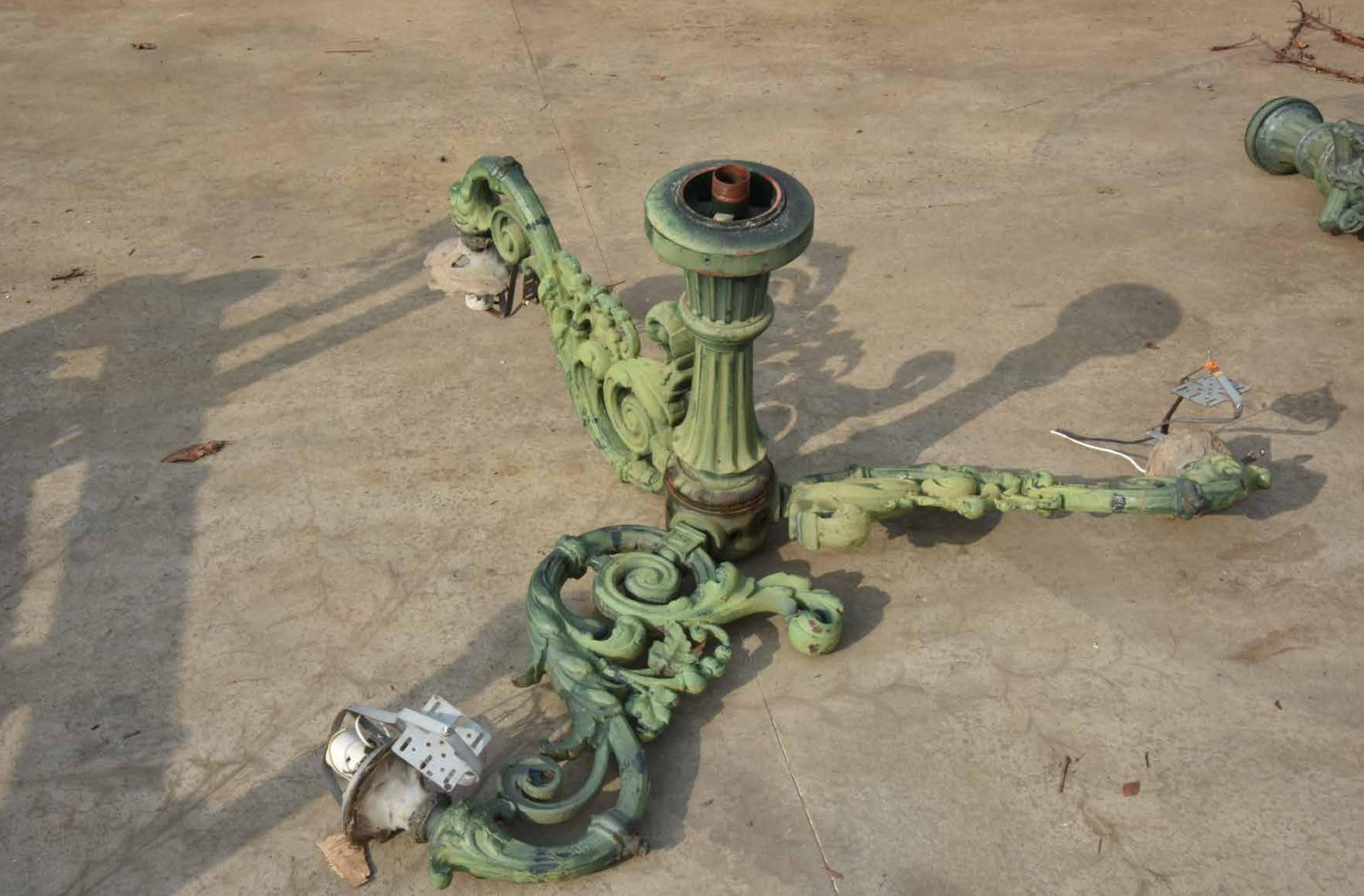
At Neri, all of the castings were carefully sandblasted to allow the disassembly of the individual elements and to highlight the damaged parts.
