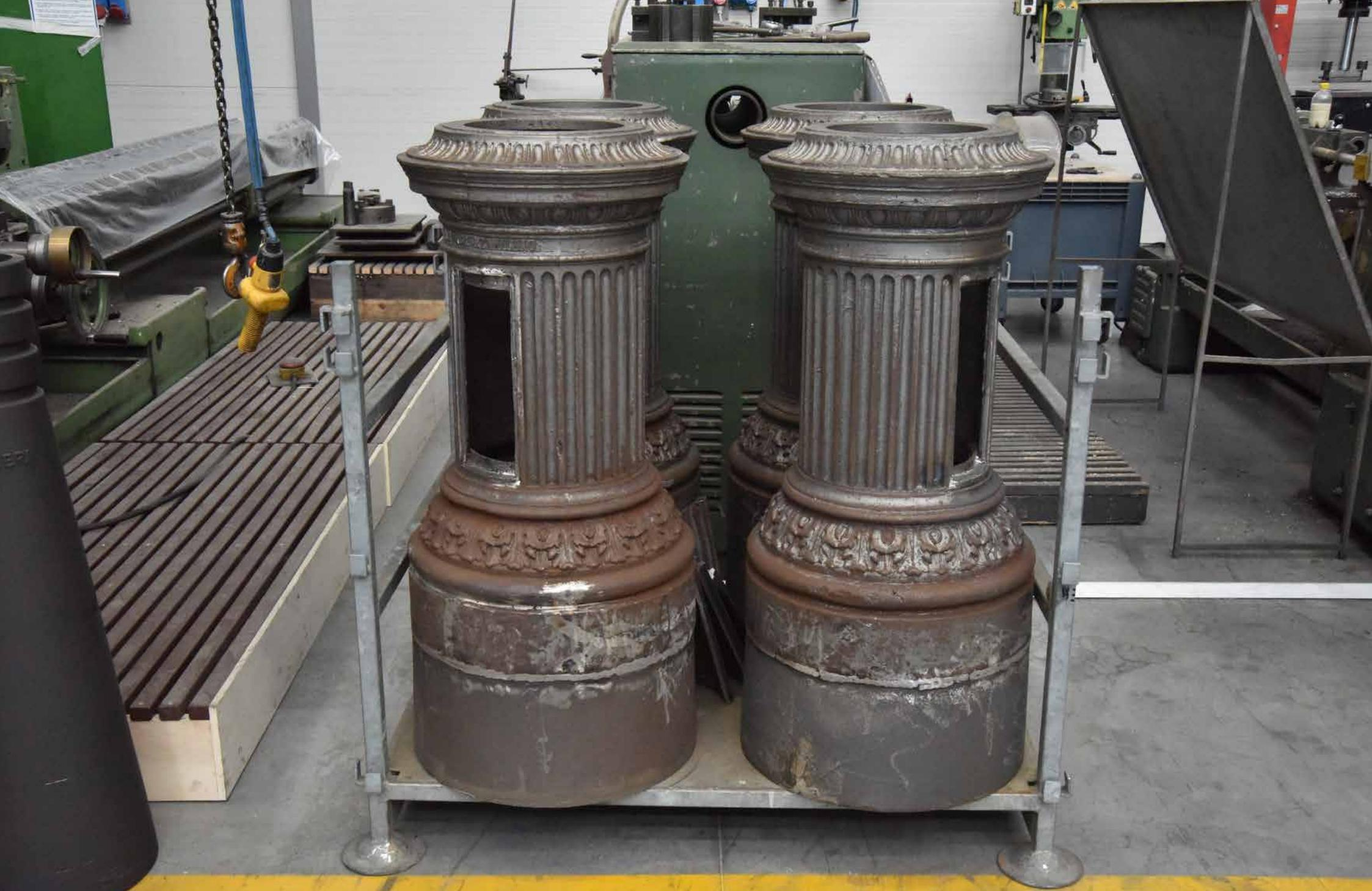
The columns, which had already been severely damaged in the past, were reinforced over time with various steel pipes inserted in them to improve the by then compromised mechanical resistance. At Neri, they were freed and given new pipes specifically calculated to guarantee maximum safety and stability.
