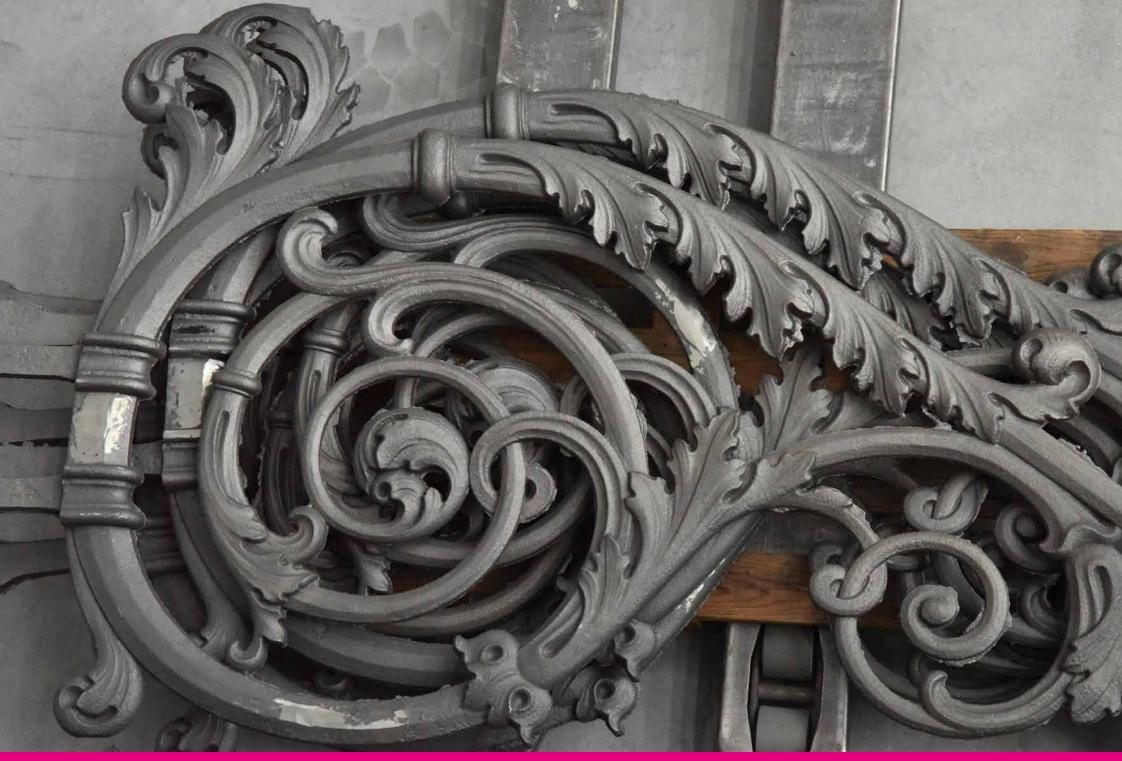
Finally, the wall brackets were carefully stuccoed and painted with two protective base coats followed by a finishing coat in Neri Grey.
