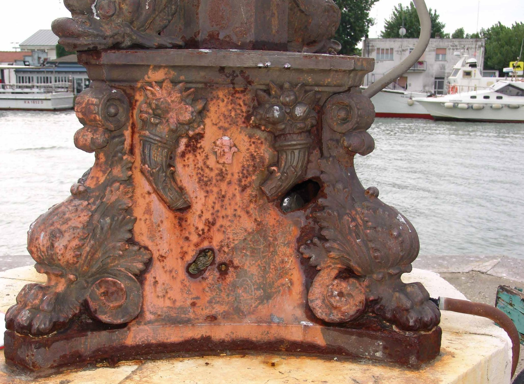
Thanks to an intervention by the Port Authority and the support of the Bank of Ravenna and Casa Matha, the lamp posts were restored by Neri SpA. In particular, the broken column was the most worrying part, because it was detrimental to the stability of the post. The column was welded and reinforced with a steel core. All parts were cleaned and the missing decorations were replicated.
